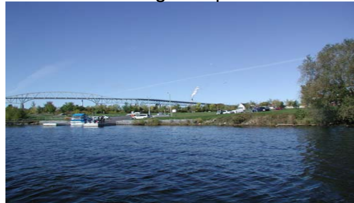
Cornwall Bridge- Exposed Zone
